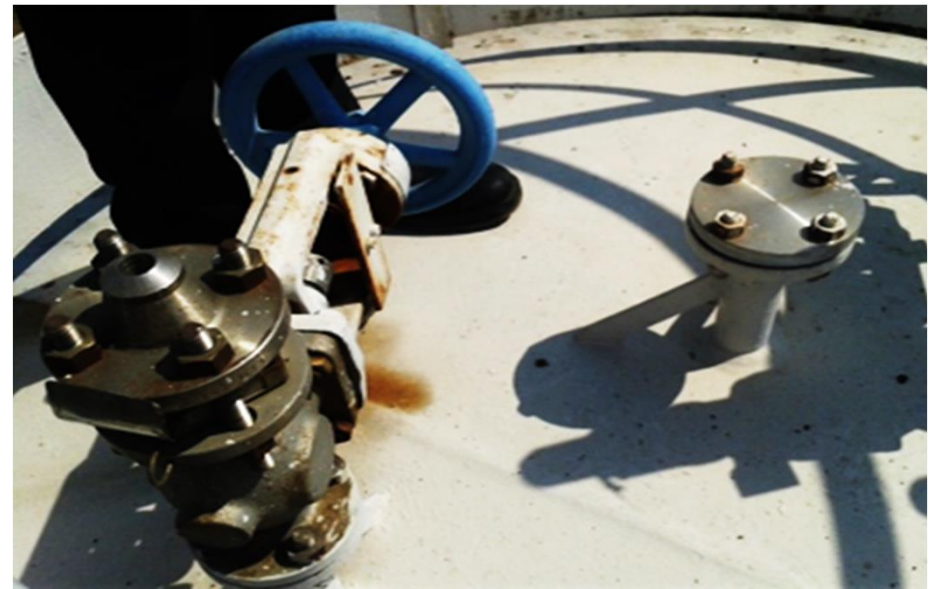
Rupture disc on high pressure helium gas vessels
