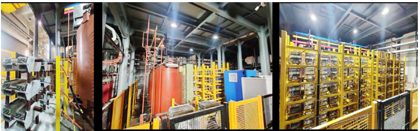
Figure B.11. The 55kV, 6MW MHVPS installed at ITER-India Power Supply Lab
