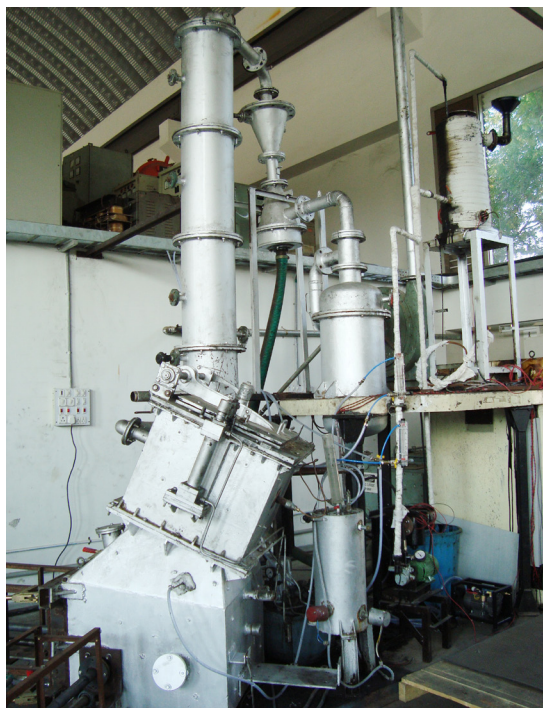
Figure B.1.1.5 Photo of the plasma pyrolysis system that is used for the pyrolysis/gasification of the petroleum residue
