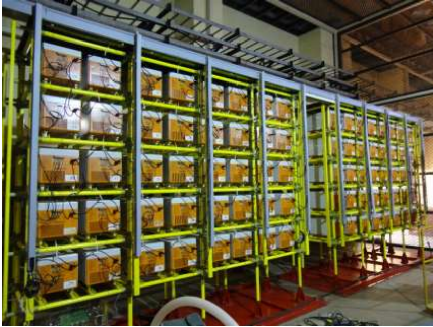
Fig. 7: Photograph of RHVPS with power modules in stacks.
