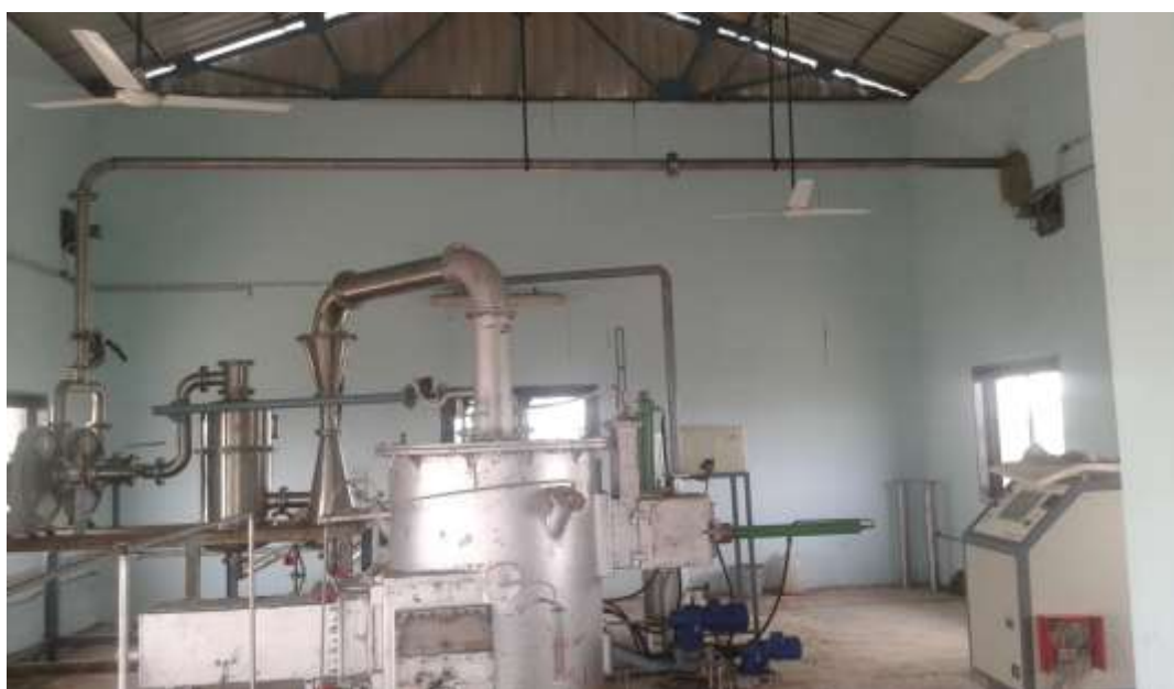
Fig. 3: Plasma pyrolysis /gasification system for the disposal of solvent waste commissioned at CSIR-CSMCRI, Bhavnagar, India.
