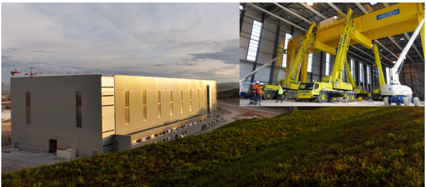
Figure B.2.2 Cryostat Workshop at ITER site, Cadarache, France and crane installed inside
