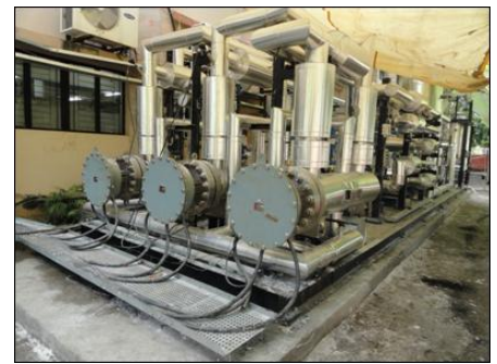
High Pressure High Temperature Water Circulation System (60 bar, 160C, 300 lpm)
