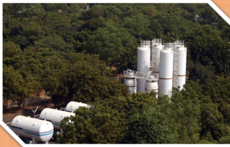
View of the liquid nitrogen and liquid helium tanks of the SST 1 cooling system - Photo by K. K .Mohandas
