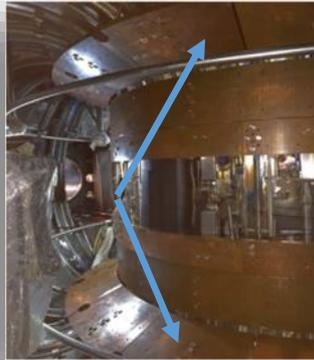
**Top & Bottom Main baffle back plate installed in SST-1 Vacuum Vessel**
