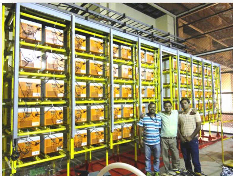
(L) The HV power supply during installation at BARC. (R) The HV isolator and ground switches of the system
