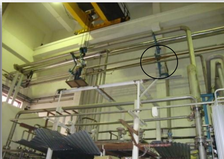
The location of the leakage in the section of LN 2 transfer Line, and the repaired LN 2 line.
