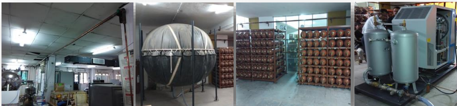
(L-R) Helium Recovery Line, Helium Gas Bag (Volume: 10\text{ m}^3 ), Stagnant Type Cylinder Bank (STCB) with 96 cylinders in total and Helium Recovery Compressor (Capacity: 20\text{ m}^3/\text{hr} )
