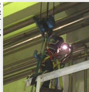
Welding in progress
