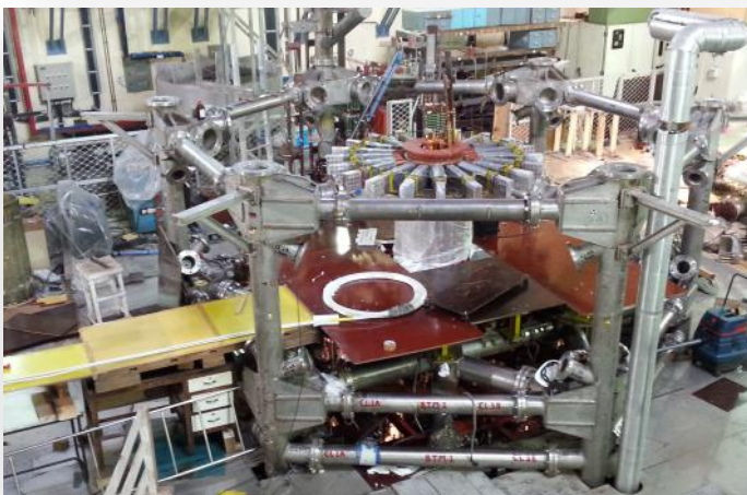
Different views of the Aditya vacuum vessel being installed. One half of the vessel as well as the inner section of the coils have been mounted.
