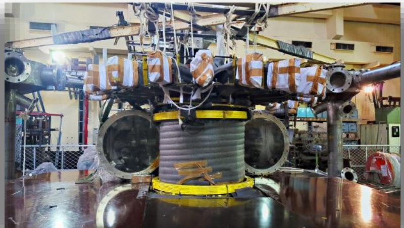
Different views of the Aditya vacuum vessel being installed. One half of the vessel as well as the inner section of the coils have been mounted.
