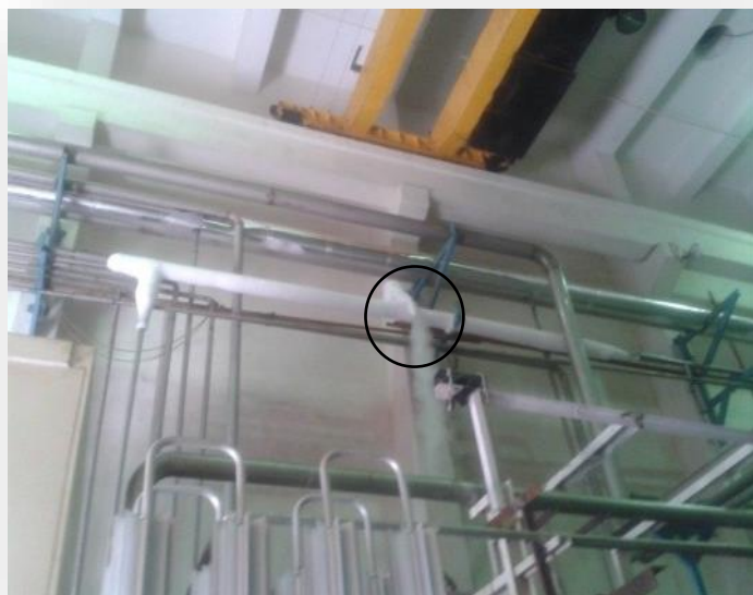
The location of the leakage in the section of LN 2 transfer Line, and the repaired LN 2 line.
