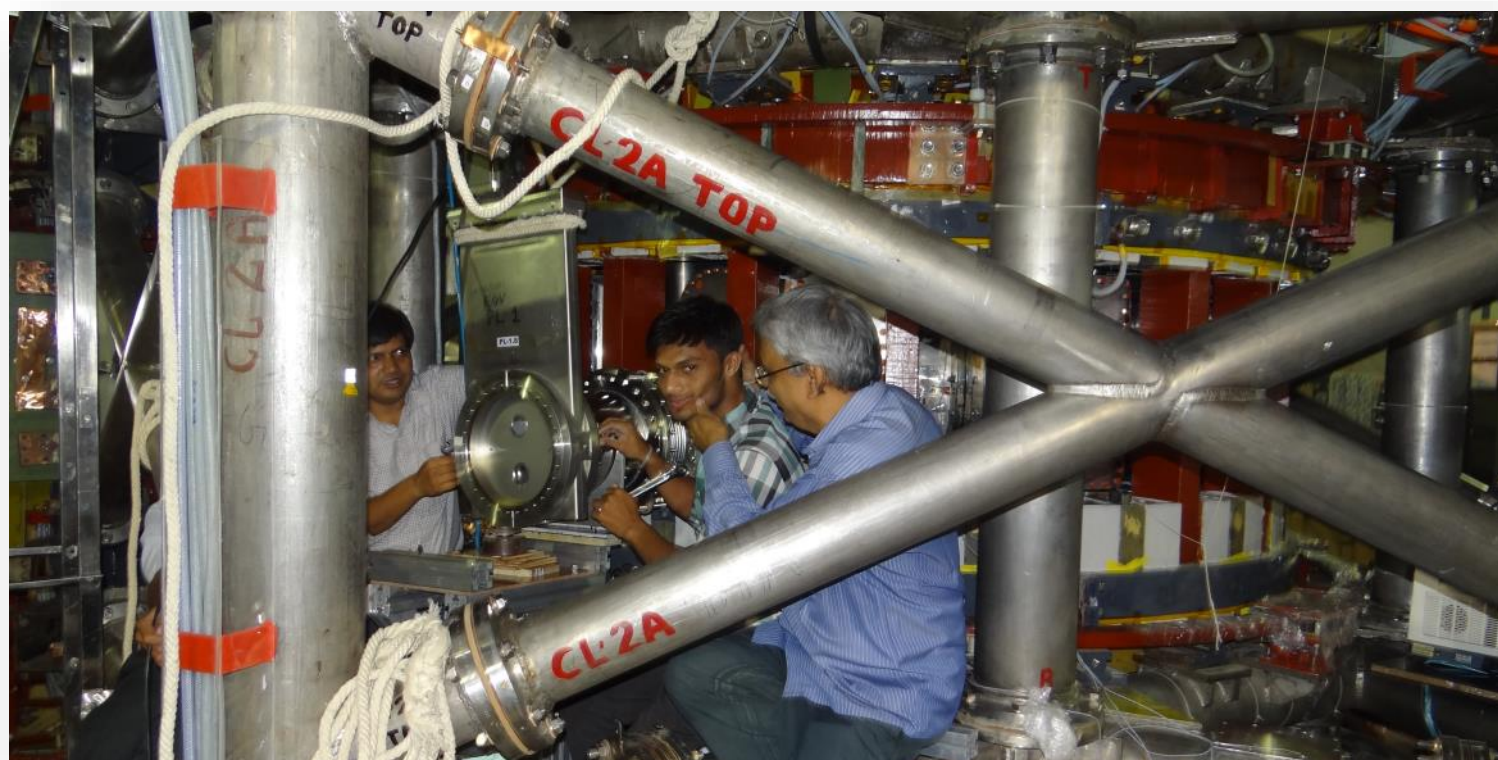
Installation of one of the gate valves on the pumping line # 1 in progress.
