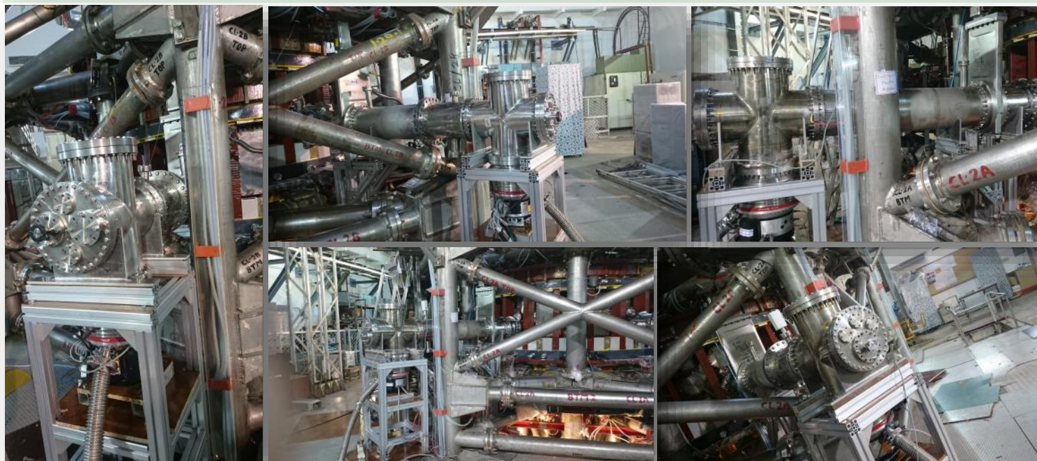
The pumping lines PL1 and PL3 and turbo-molecular pumps installed on the Aditya-U device
