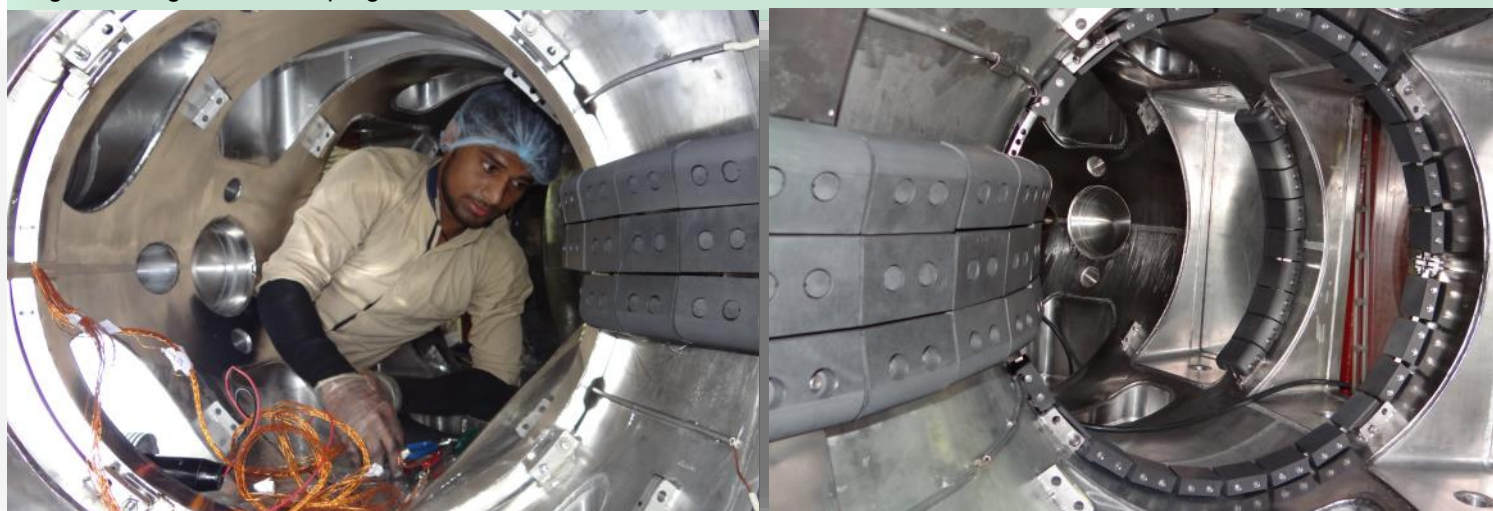
Installation of the inner toroidal and the outer poloidal limiter in progress inside the Aditya vessel.
