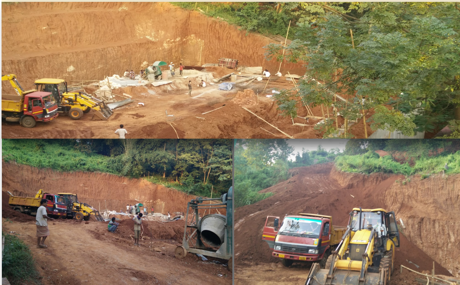
construction of Canteen building and site grading works started at CPP-IPR
