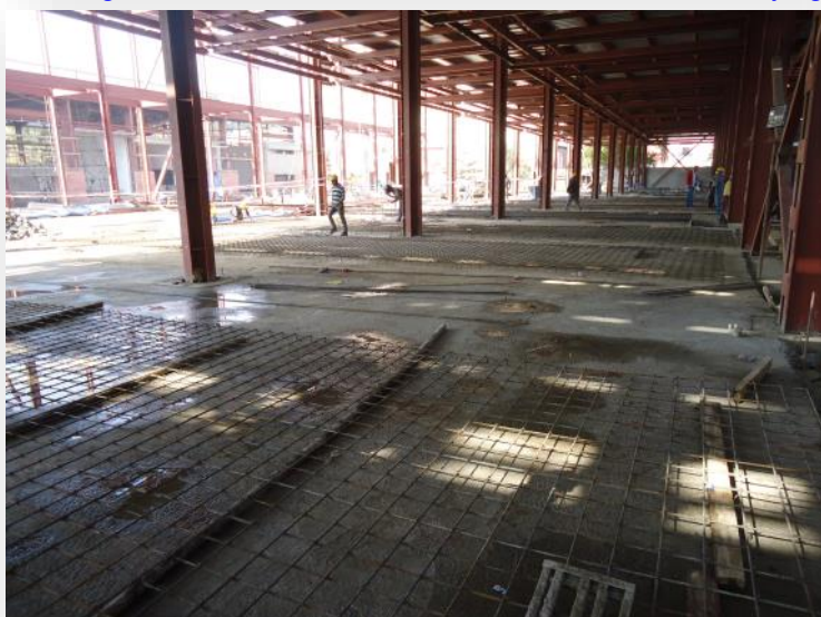
(Left) View from inside the laboratory building (below Mezzanine floor) showing the Tremix flooring reinforcement work in progress. (Right) View from ITER building side of the tower column erection for the laboratory building.
