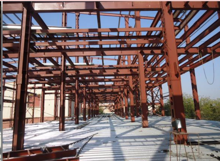
(Left) View from inside the auxiliary showing the completed Tremix flooring (Right) View from inside the laboratory building at 7.5m level on the mezzanine floor. Work for laying RCC slab at this level is in progress.
