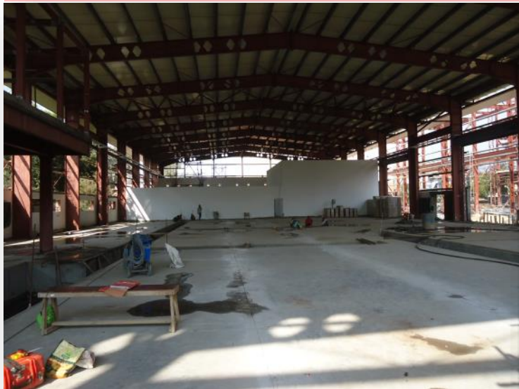
(Left) View from inside the auxiliary showing the completed Tremix flooring (Right) View from inside the laboratory building at 7.5m level on the mezzanine floor. Work for laying RCC slab at this level is in progress.
