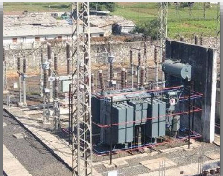
Images of the newly installed Andrew Yule make transformer at IPR switchyard
