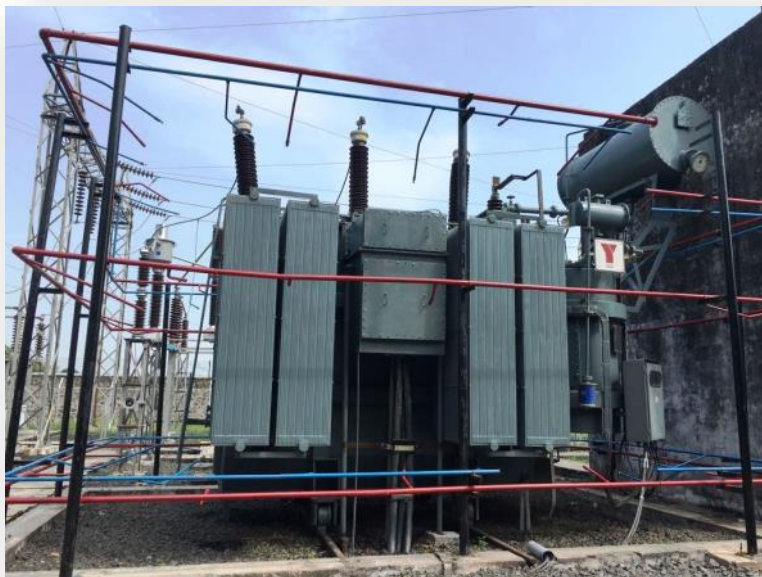
Images of the newly installed Andrew Yule make transformer at IPR switchyard
