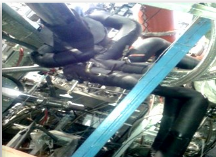
Flexible Elastomer Foam Nitrile Insulation on SC duct piping and surfaces at 80 K Temp
