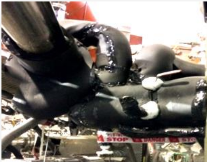
Flexible Elastomer Foam Nitrile Insulation on SC duct piping and surfaces at 80 K Temp
