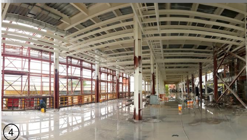
(1) The laboratory building roofing work in progress (2) Roofing work in progress, as seen from 2nd floor of the laboratory building (3) View of the auxiliary building from the control room showing the water chiller piping installation being carried out. (4) Fire-retardant painting of the beams in the 1st floor of laboratory building. (5) View of the high-bay area of the laboratory building from the 2nd floor.
