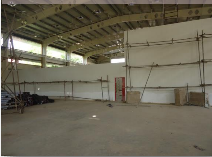
(L) Inside the auxiliary building showing the control room partition. (R) The cooling stations outside the auxiliary building.
