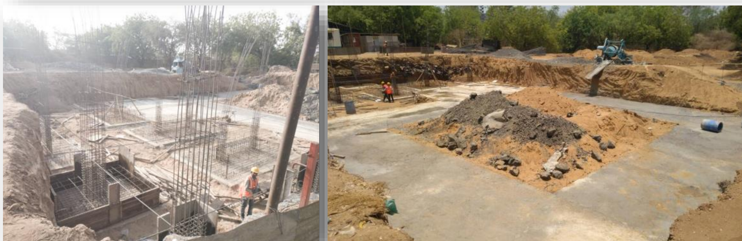
The construction of the Neutronics Laboratory : (L) Footing steel work (R) PCC work in progress
