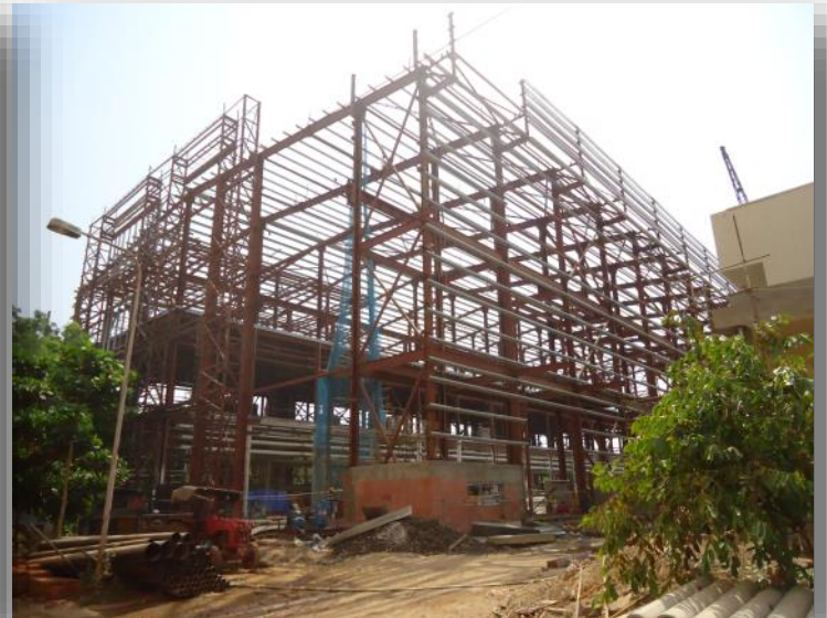
(L) The transformer bays in the auxiliary building. (R) Erection of Roof Purlins and side runners in progress in the laboratory building.
