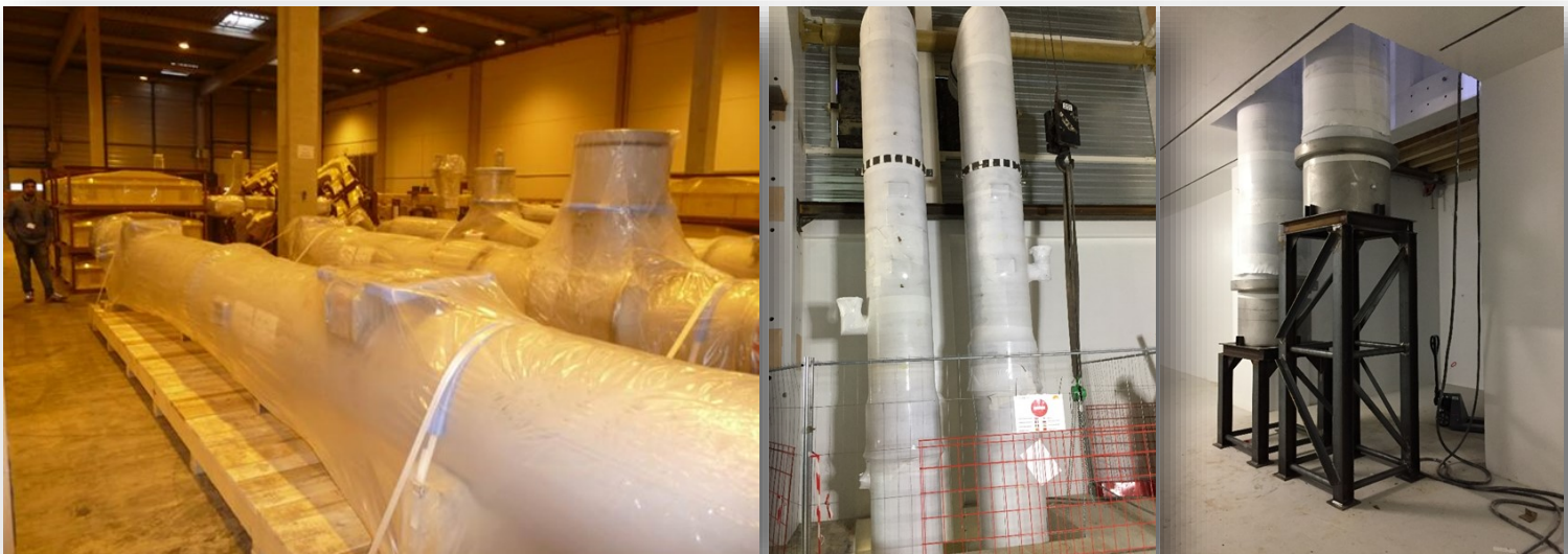
(L-R) Delivery and incoming inspection of Group X3 Cryolines and Installation of two spools of Y-group Cryolines at ITER site at ITER France
