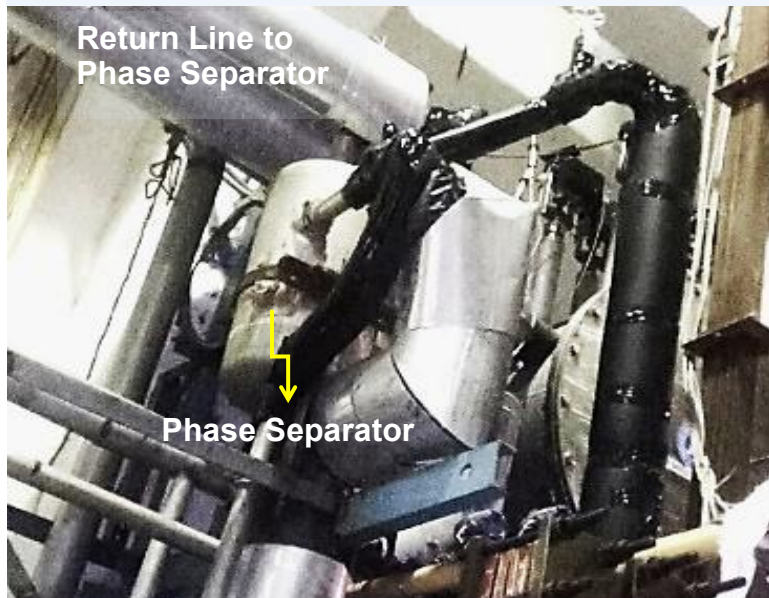
(L) Re-routed insulated line to 15 L phase separator (R) LN 2 flow rate measurement in 50 L Dewar
