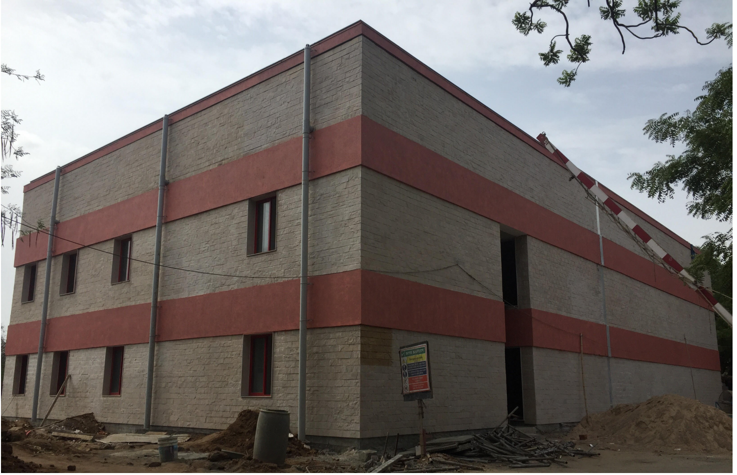
The completed external stone cladding of the Neutronics Laboratory
