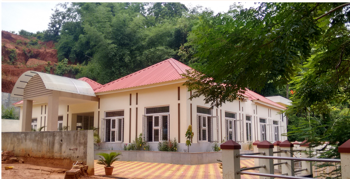
View of the new canteen building
