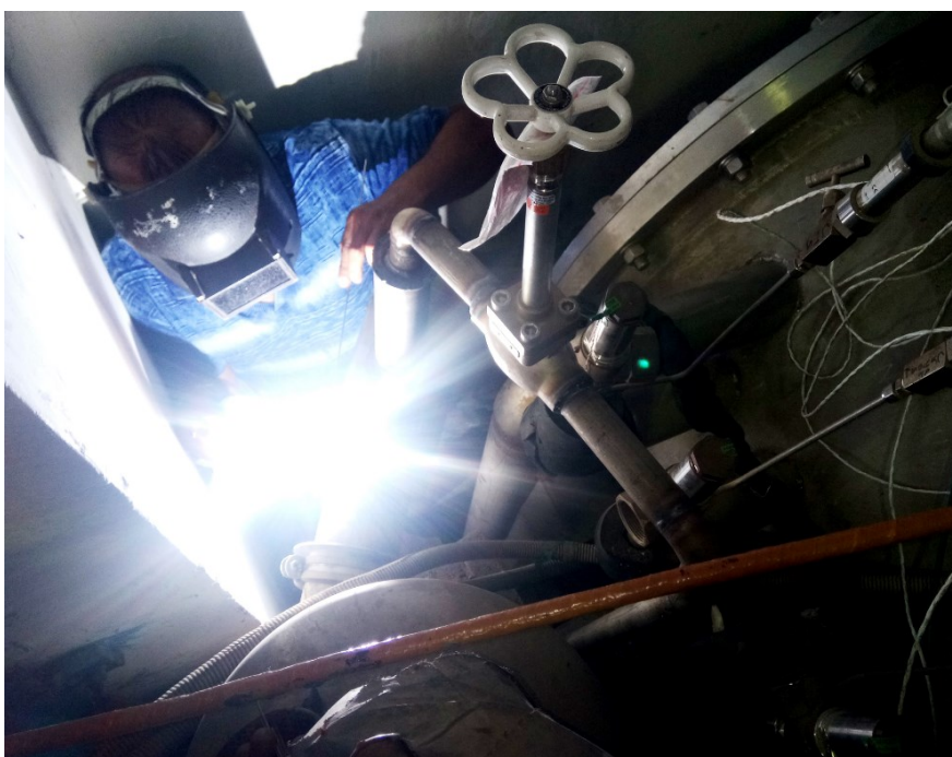
(L) Welding of 80 K Return Lines to LN2 Phase Separator (R) Dye penetration NDT test of the line
