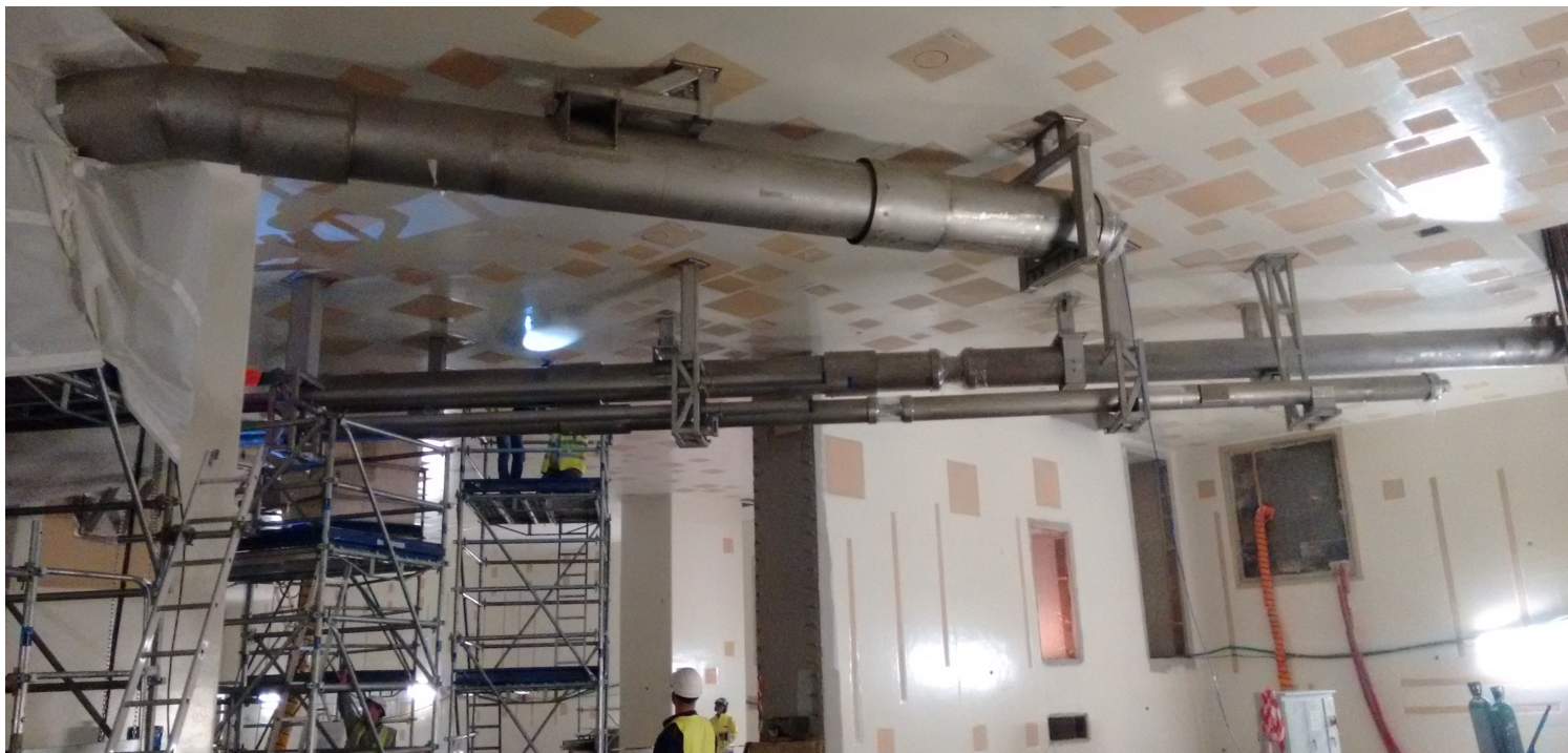
Cryo-line positioned in its final location supported through embedded plates of the building
