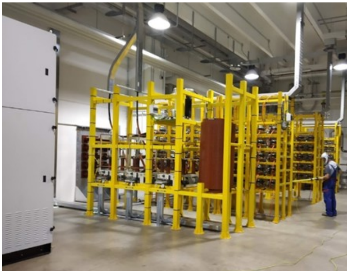
(L) Installed AGPS at SPIDER facility (R ) AGPS voltage and current waveforms along with RF and extraction voltage
