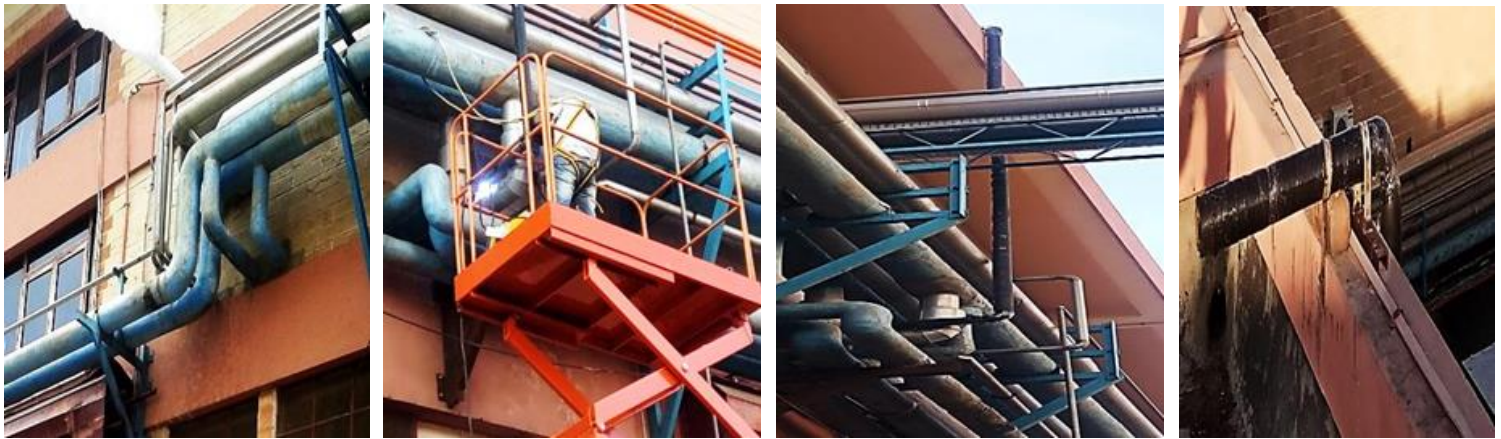
(L-R) LN 2 Liquid/vapour venting out, Welding of the line. Extended thermal insulated LN 2 vent lines
