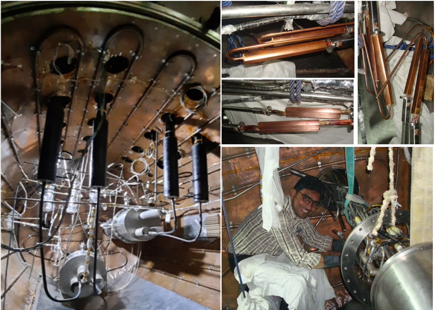
(L) The installed and insulated current leads and sensors in FSC (Top) A pair of fabricated coil and current lead lap joint (Bottom) Welding job in progress
