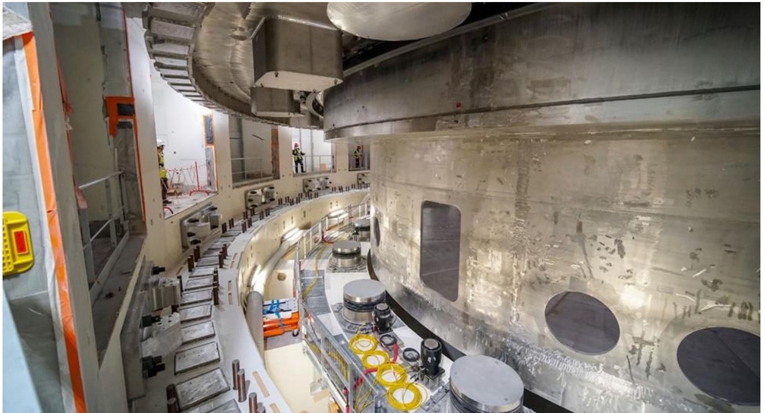
Cryostat Base Section positioned in the Tokamak Pit
