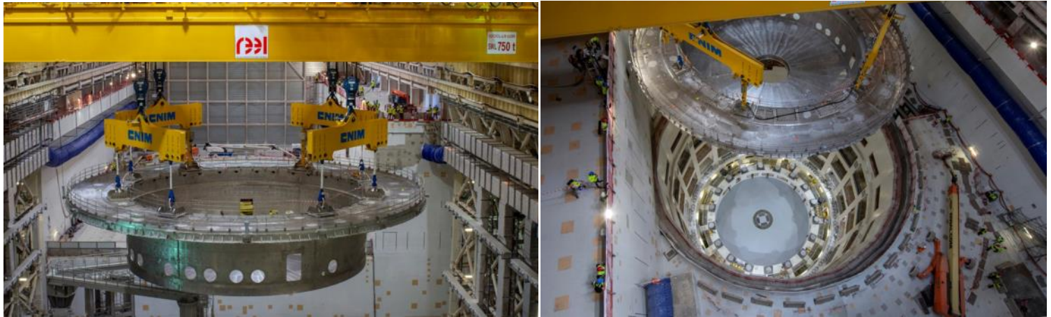
(L) Lifting Operation of Cryostat Base Section, ~1250 tons (R) Cryostat Base Section being lowered in the Tokamak pit
