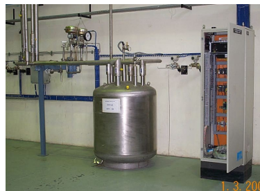
Figure 3 Photographs of LN 2 Storage system along with Sub-cooler Dewar at Cryo Hall
