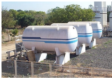
Figure 3 Photographs of LN 2 Storage system along with Sub-cooler Dewar at Cryo Hall
