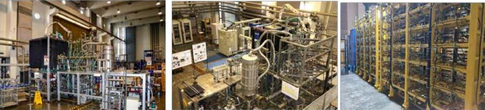
The commissioned 6 MW main high-voltage power supply for the gyrotron cathode circuit at ITER India.
