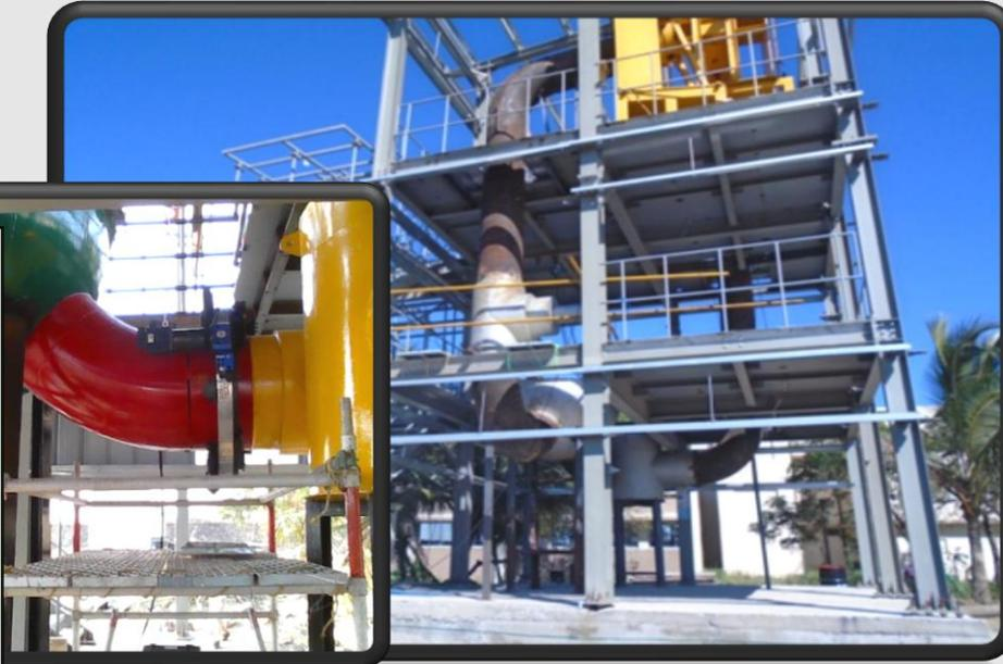
*Full Scale Mock-up for Reactor 24 Inch Recirculation Pipe Line*
