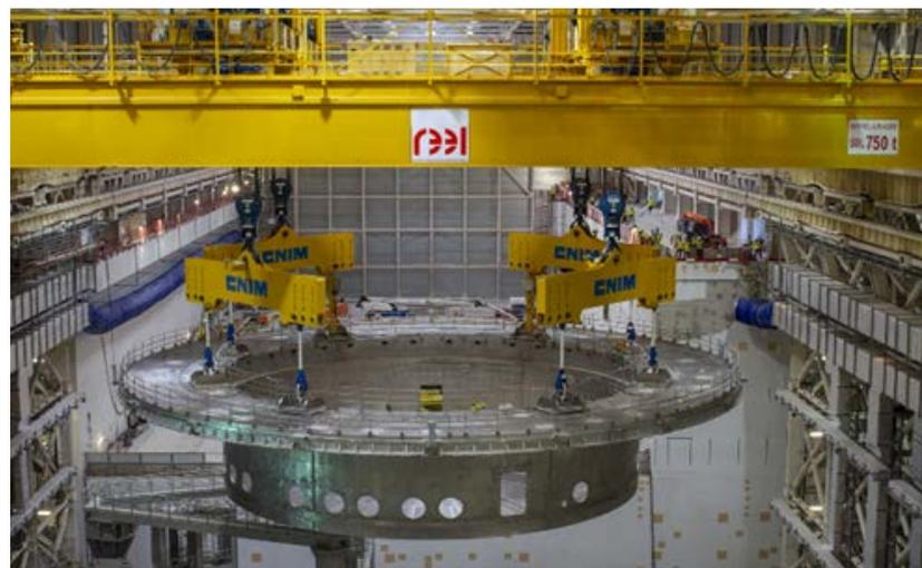
**Lifting Operation of Base Section in Tokamak Pit**
