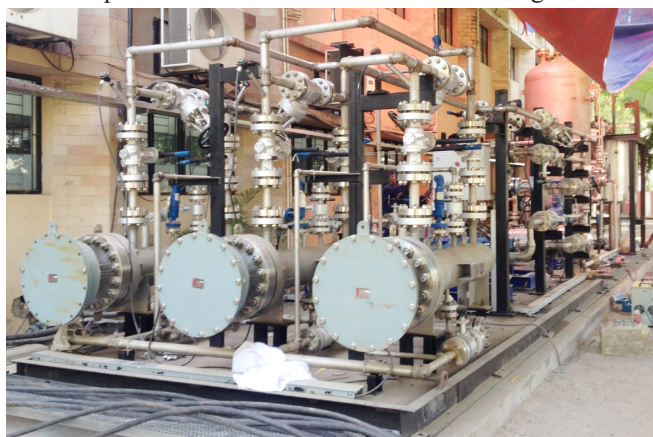
Figure A.2.3. High Pressure High Temperature Water Circulation System (HPHT-WCS) for HHFTF
