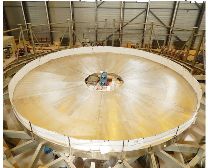
Figure B.2 Cryostat Base Section Tier-1 welding and testing at ITER site workshop
