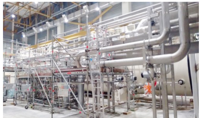
Figure B.8 Installation of warm lines and cryolines underway at ITER site
