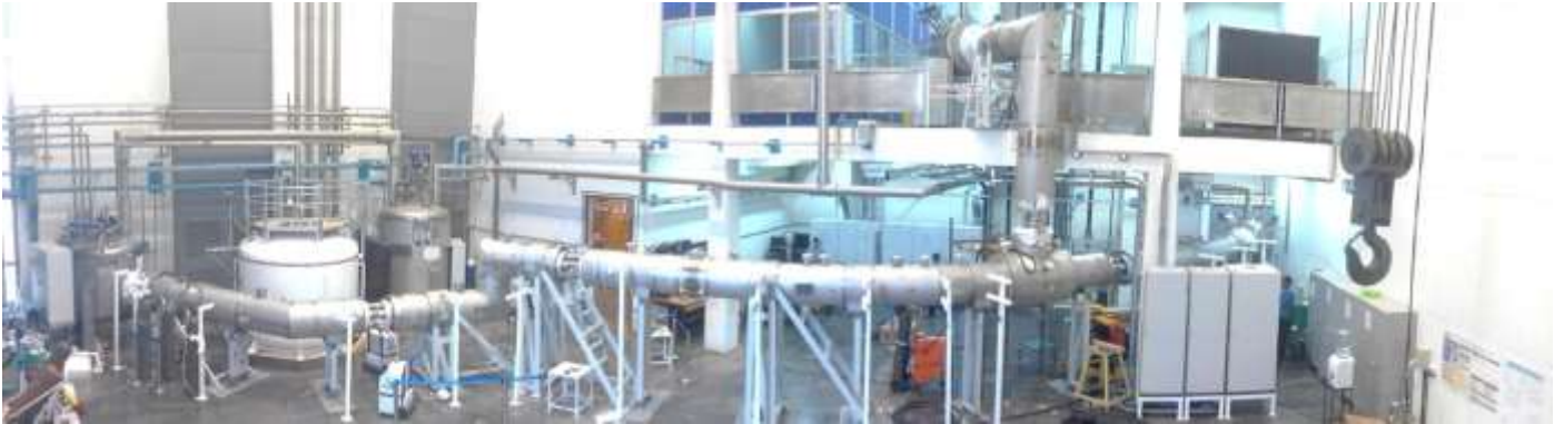
Figure Prototype Cryoline Installed at ITER-India Laboratory, Completion of Thermal Cycling test from 300 K to 4.5 K, three times.
