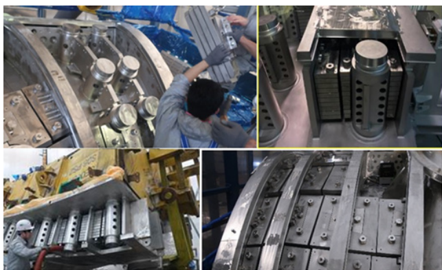
Figure B.1.4: In sequence : IWS lowered for assembly in VV sector; IWS assemble around flexible support housing between outer and inner shells of VV, inspection after assembly to ascertain needed clearance, VV segment view after assembly of IWS and ready for welding the outer shell.
