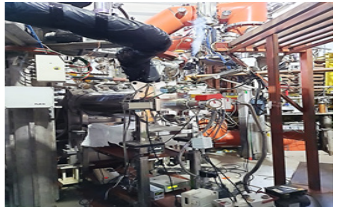
Figure A.4.13: Sorption pump installed on the radial port of the SST-1 Tokamak.
