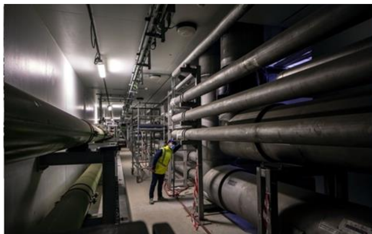
Cryolines and Warmlines manufactured by M/S INOXCVA under installation at ITER site
