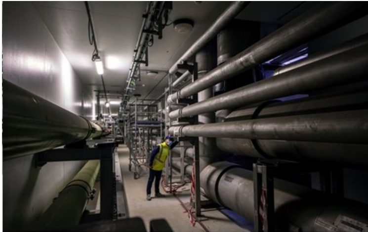
Cryolines with multi feed pipes supplied by India under installation at the ITER site
