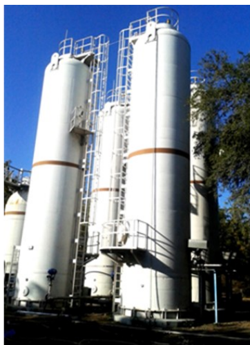
(L-R) : High pressure and medium pressure storage vessels; Hydro test pressure @ 203.5 bar (g) and at 23.4 bar (g)
