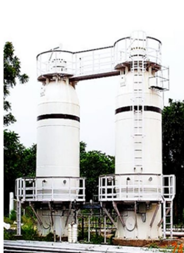
(L-R) : High pressure and medium pressure storage vessels; Hydro test pressure @ 203.5 bar (g) and at 23.4 bar (g)
