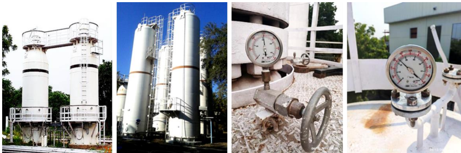
(L-R) : High pressure and medium pressure storage vessels; Hydro test pressure @ 203.5 bar (g) and at 23.4 bar (g)
