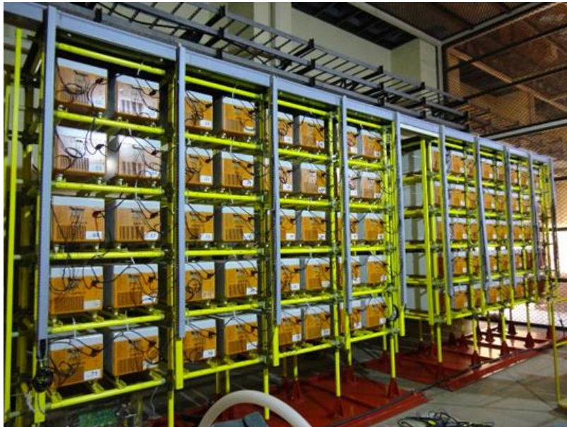
100kV, 25 A Regulated High Voltage Power Supplies (RHVPSs) installed at BARC site. Waveform shows 80kV application by RHVPS at repetition rate of 2Hz to Klystron cathode
