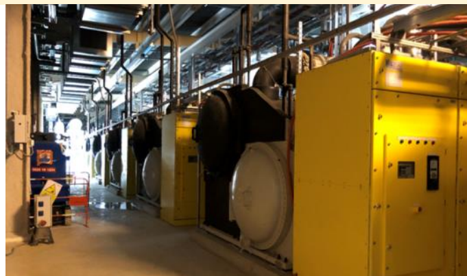
(L) The installed cooling tower (R) Installed chillers and soft starters
