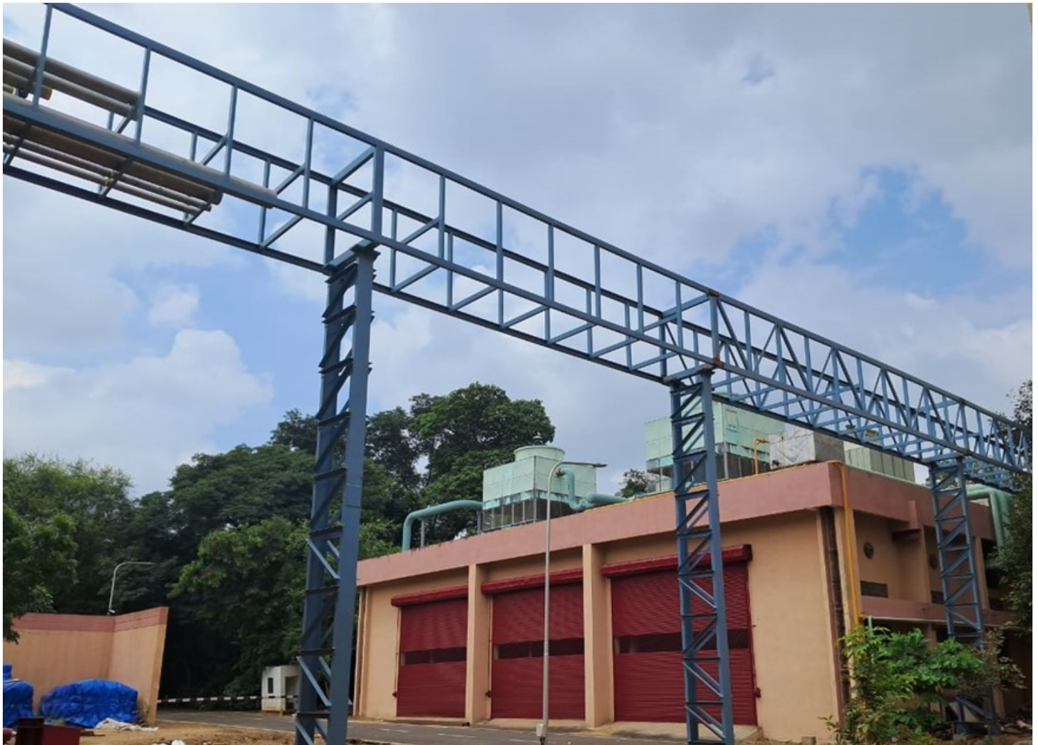
Piping supports for the CWS for ITER-India & IPR Labs under construction at IPR main campus
