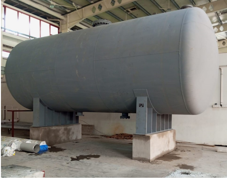
(L) Storage tank installed in the plant room (R) Concrete pedestals
