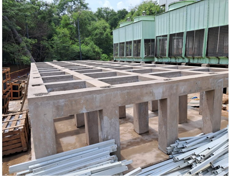
(L) Storage tank installed in the plant room (R) Concrete pedestals
