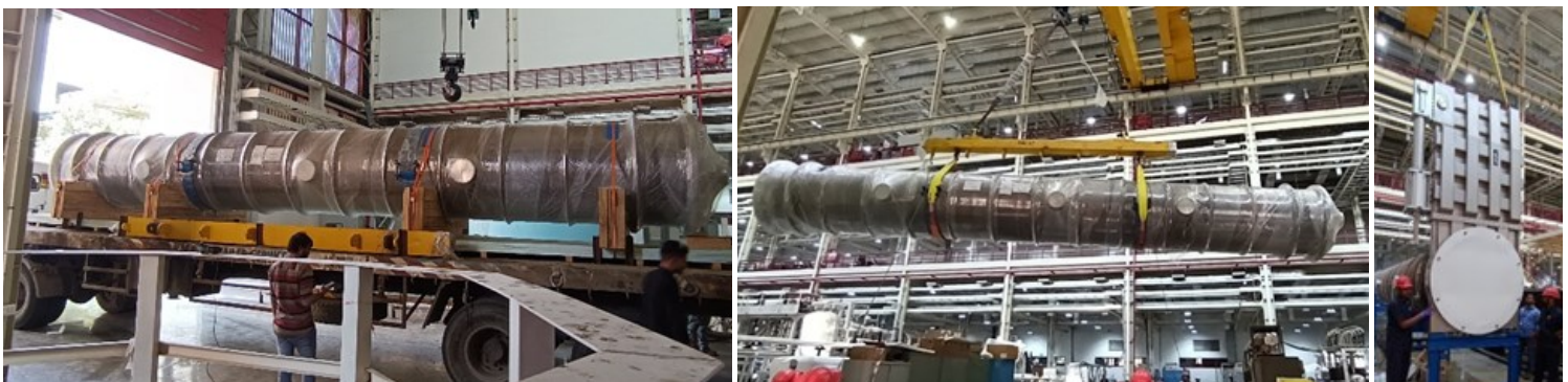
The vacuum vessels and the gate valve assembly being unloaded at IPR New Laboratory Building
