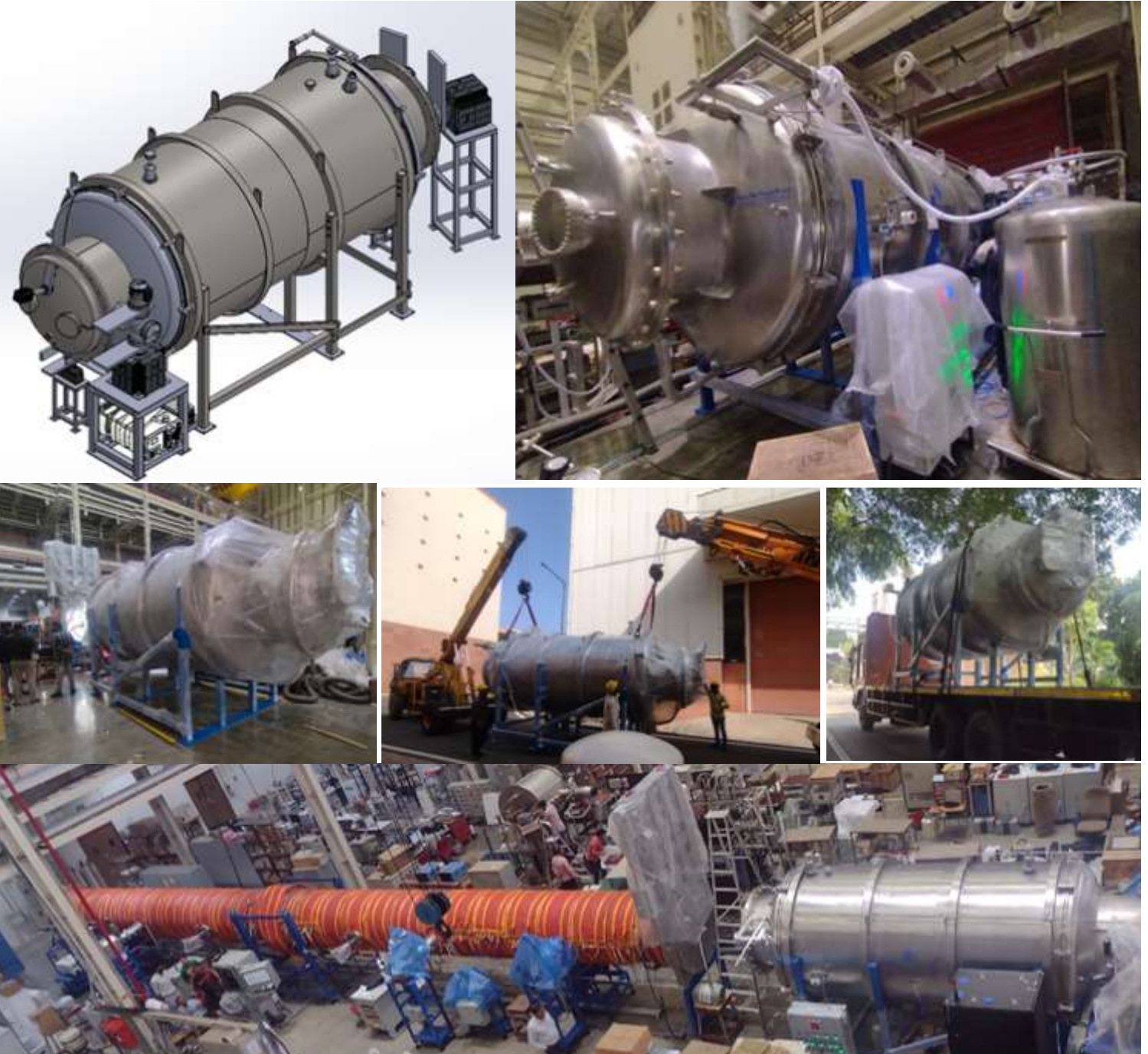
Images of the installation of the cryo-pump for the LIGO-India VISTA facility at IPR
