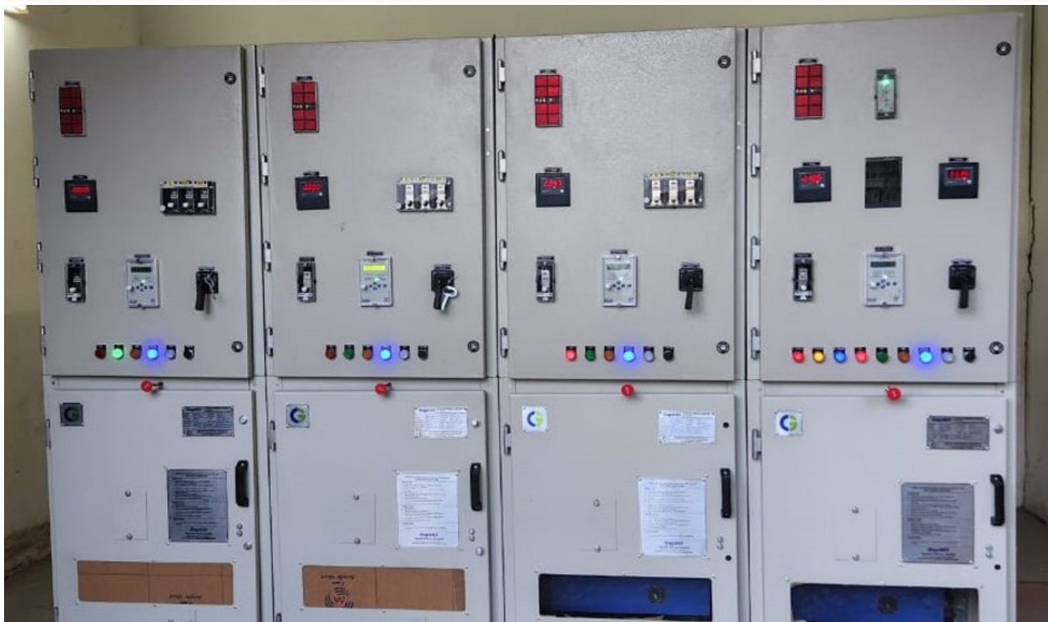
The new 11kV HT Panel installed at FCIPT
