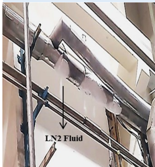
LN2 leakage in main vent line
