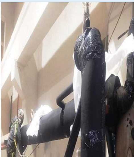
Thermal insulation installation process
