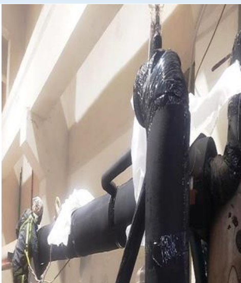
Thermal insulation installation process
