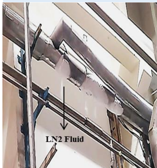
LN2 leakage in main vent line
