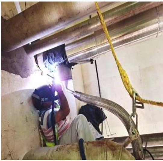
Phase separator assembly in 80 K vent line
