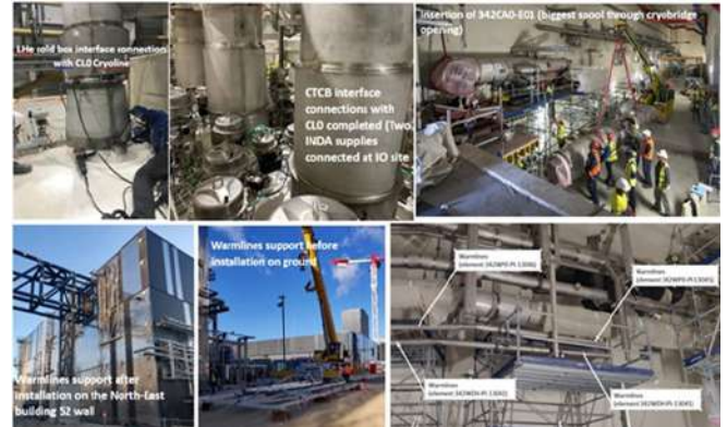
Figure B.1.5: Installation of X, Y cryolines and warmlines at ITER site.
