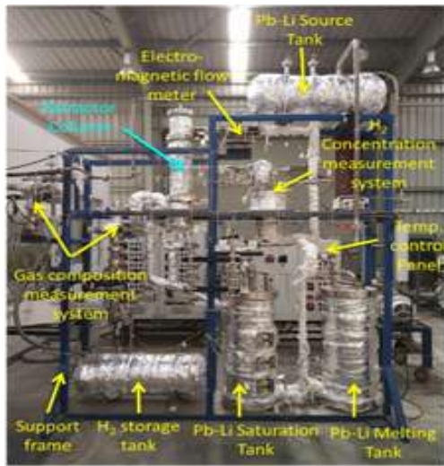
Figure A.4.12: Installed HIES set-up.
