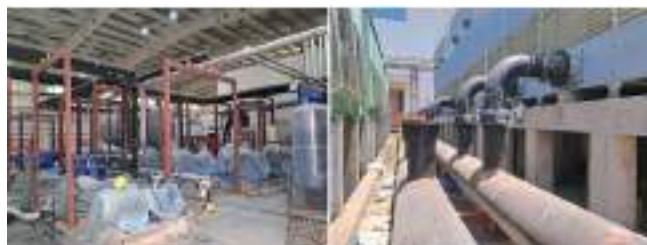
Figure A.6.1: Ongoing installation activities.
